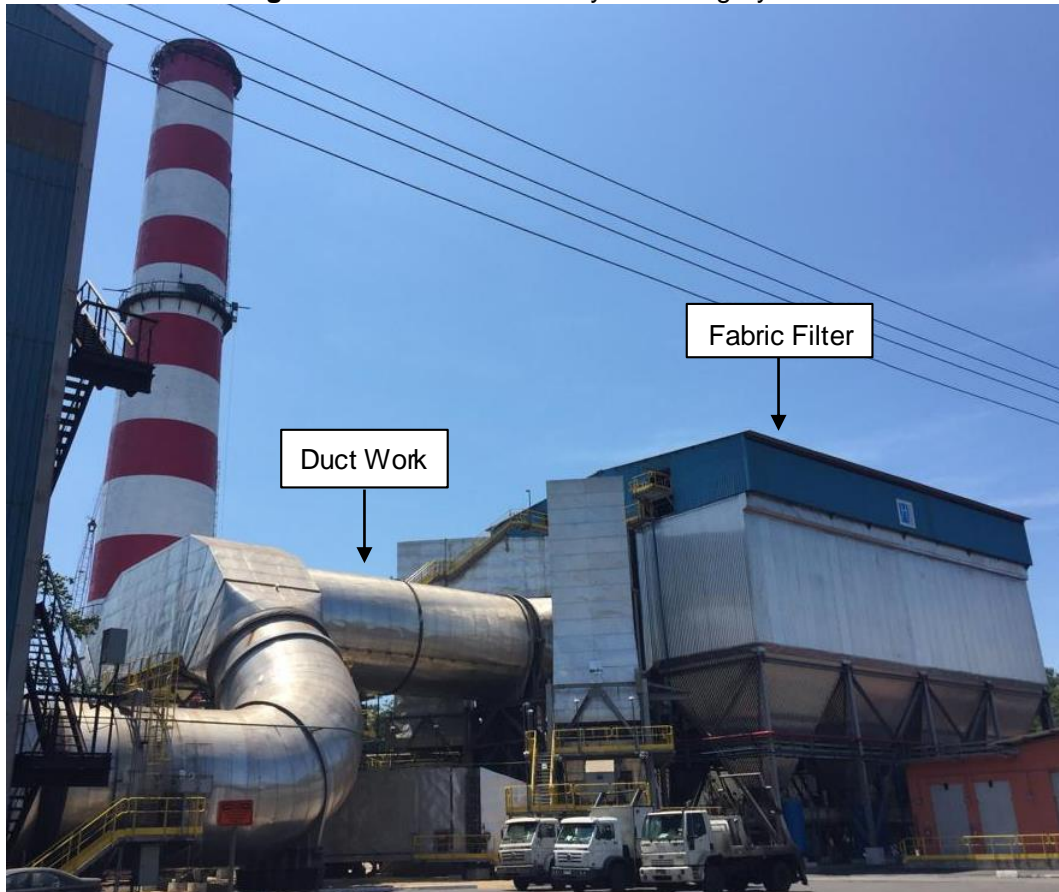
Figure 4: Sinter Plant Primary Dedusting System.
